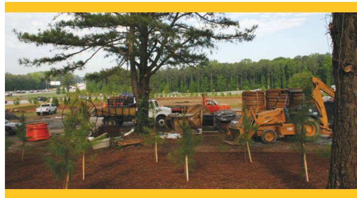
Workers remake the Haynes Bridge interchange.
