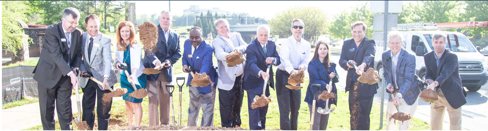
ABOVE: NFCID Board Members join North Fulton leaders in breaking ground on Windward Parkway Phase II
