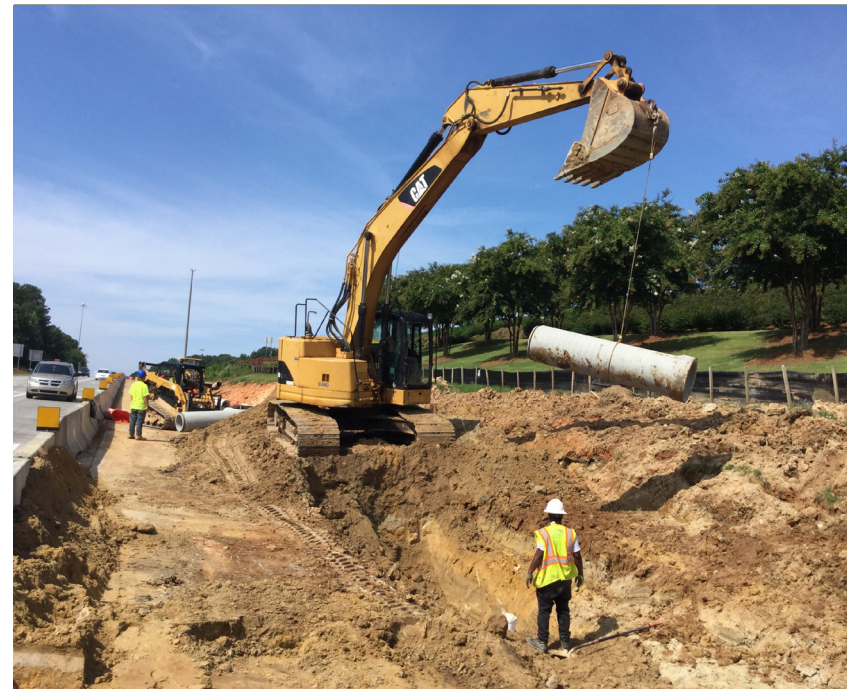
ABOVE: Windward Parkway Phase II Construction
