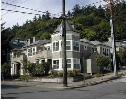
Multifamily buildings can be designed like a mansion to be compatible with large historic single family homes.
