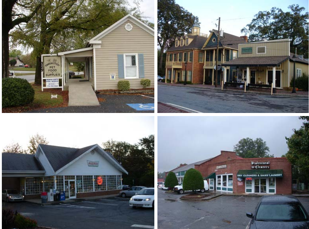
Commercial structures vary by type, size and style within the study area.
