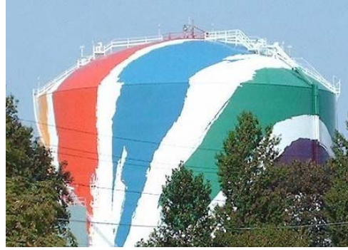
This gas tank in Boston is a regional landmark because of the work of artist Sister Corita Kent.
