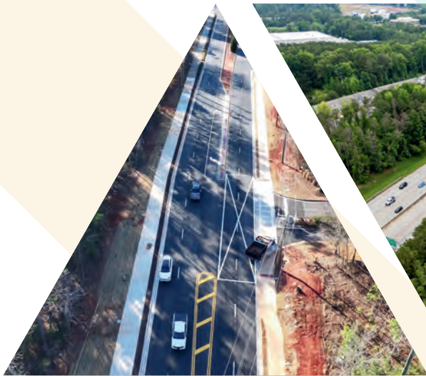
Kimball Bridge Road Gap Connection project is completed
